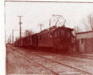
ELECTRIC SERVICE SOUTH SHORE
